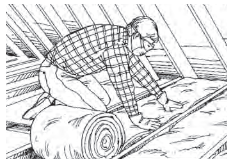
Up to 20% of your heating can be lost through your ceiling. Proper insulation can significantly cut these losses.
